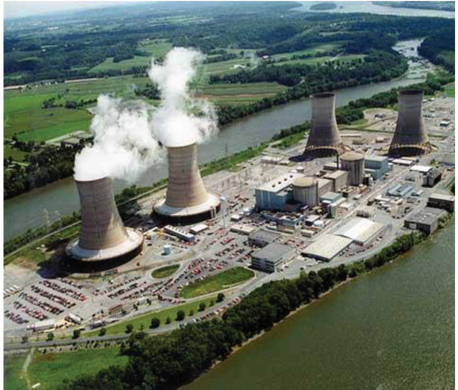
Evaporative cooling at certain types of power generation facilities represents a significant use of water in the Basin (Three Mile Island Nuclear Power Station pictured).
