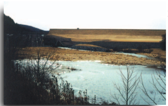
Cowanesque Reservoir Dam near Lawrence, PA.
