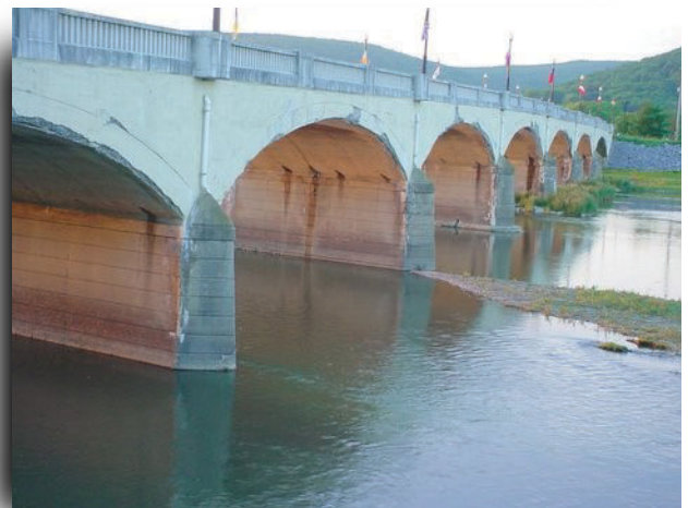
Chemung River Walking Bridge in Corning, N.Y.
