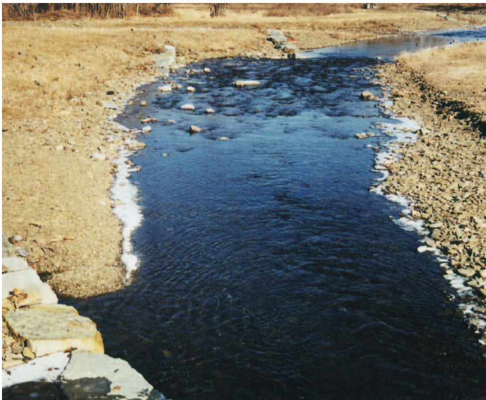
Bentley Creek stream channel restoration project near the PA/NY state line.
