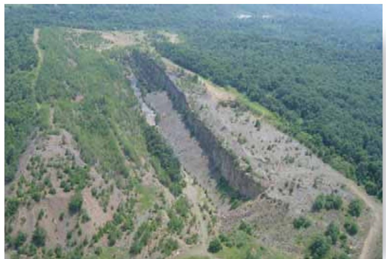
Hazardous highwall in the West Branch Susquehanna Subbasin.
