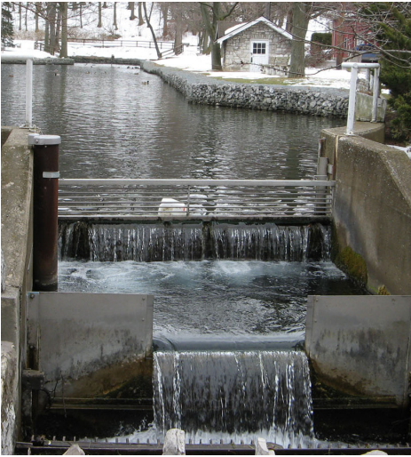
Roaring Spring outflow (instrumented weir provided daily flow measurements for use in this study).
