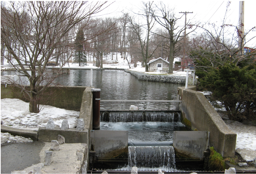
Figure 7-6. Roaring Spring Outflow (Instrumented weir provided daily flow measurements for use in this study.)
