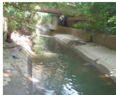
Downstream view of Paxton Creek, Dauphin Co., Pa.
