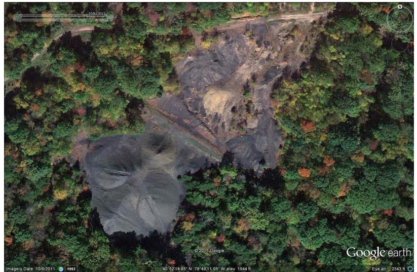
The Banks #2 coal refuse site. Keal Run coal refuse piles will be added to this site and reclaimed in total as Phase IX.
