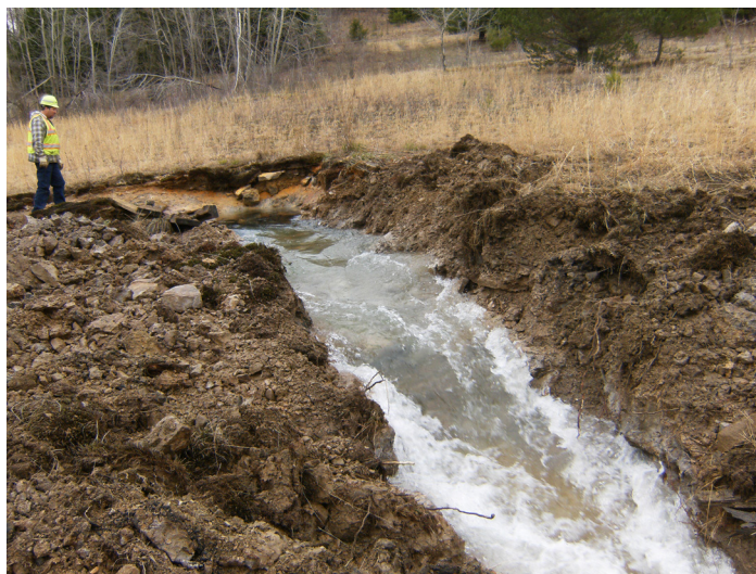
Phase IV mine pool water exiting the breach upslope of the mine seal.
