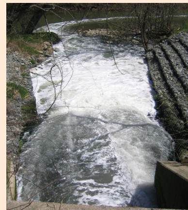
Municipal wastewater discharge point.
