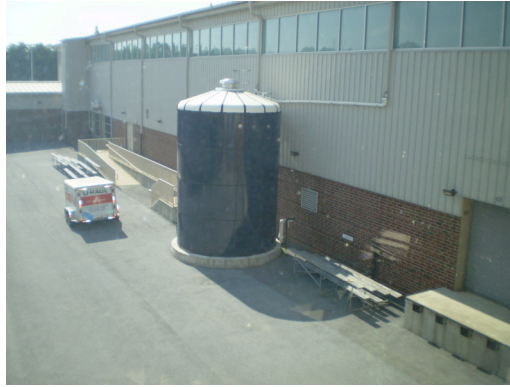
Equine Arena Roof Runoff Tank
