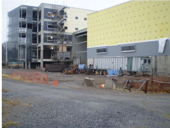
Capital View Commerce Center Under Construction in 2008
