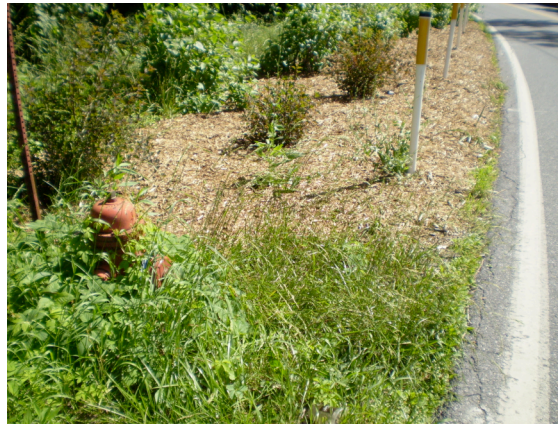
Roadside Vegetated Swale-Rain Garden
