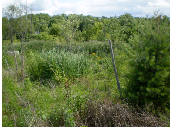
State Police Bioretention Garden
