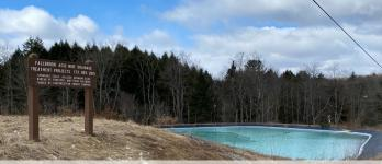
The Fall Brook facility uses three limestone beds and a polishing pond that remove toxic metals. The largely cleaned water is then released back into Fall Brook, a tributary of the Tioga River.
