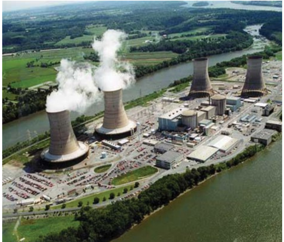
Evaporative cooling at certain types of power generation facilities represents a significant use of water in the Basin (Three Mile Island Nuclear Power Station pictured).
