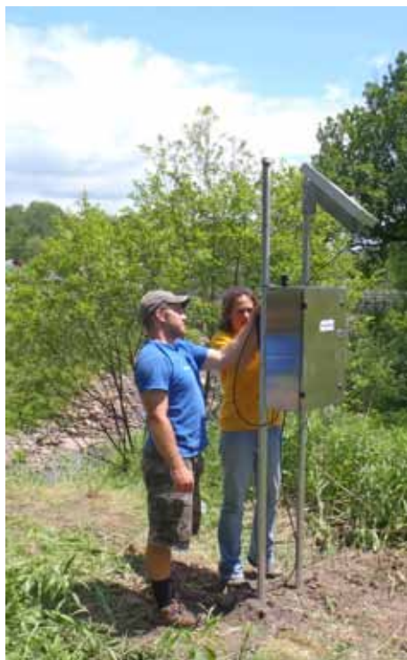
SRBC staff verifies that the station along Loyalsock Creek is working.
