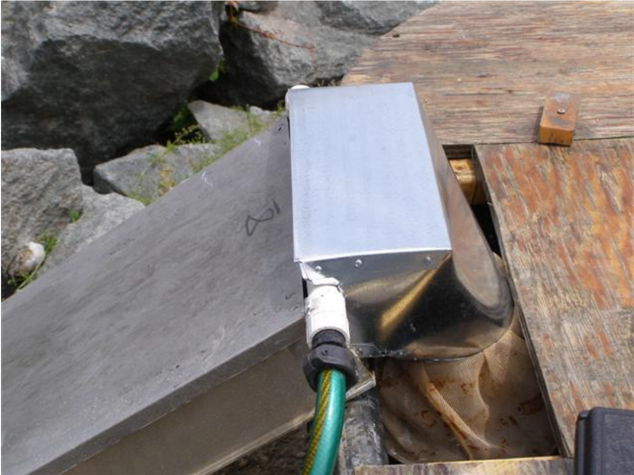
Figure 4. The cable tray emptying into a collection bag in a holding tank.
