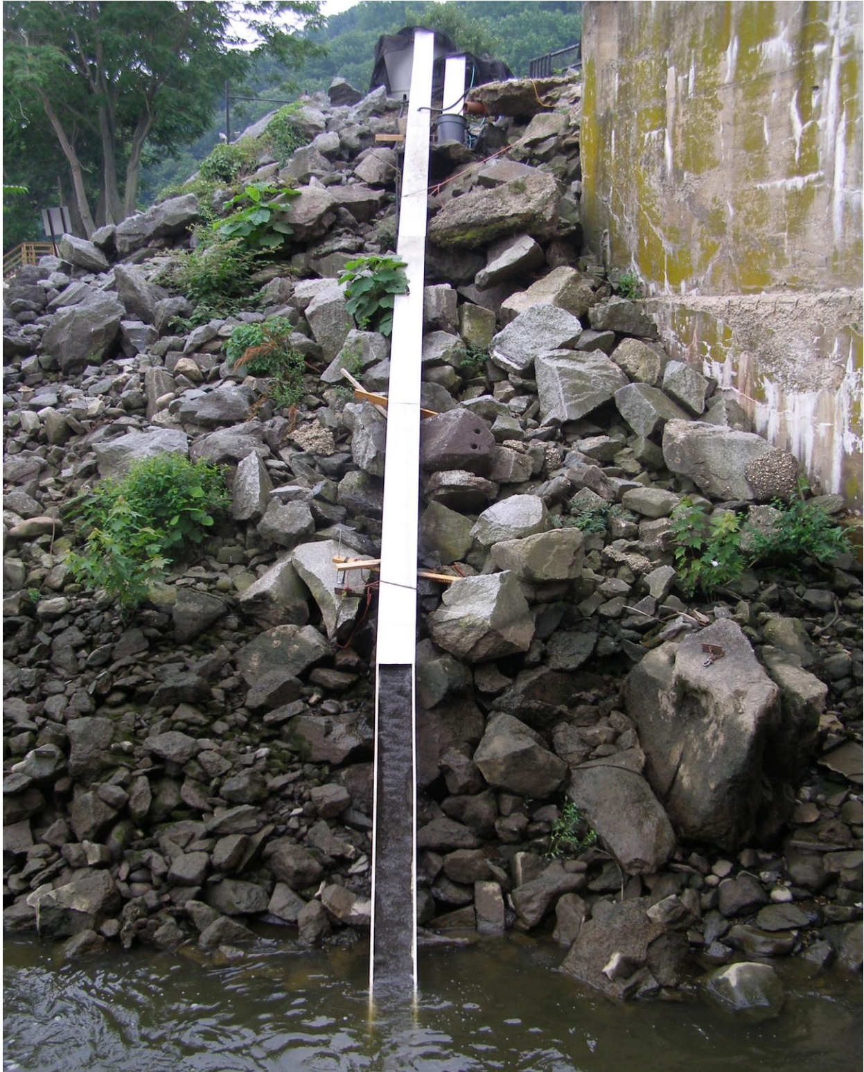
Figure 3. Cable tray on the West Shore below Conowingo Dam, tray on the left is the experimental, and the tray on the right is the control location from 2008.
